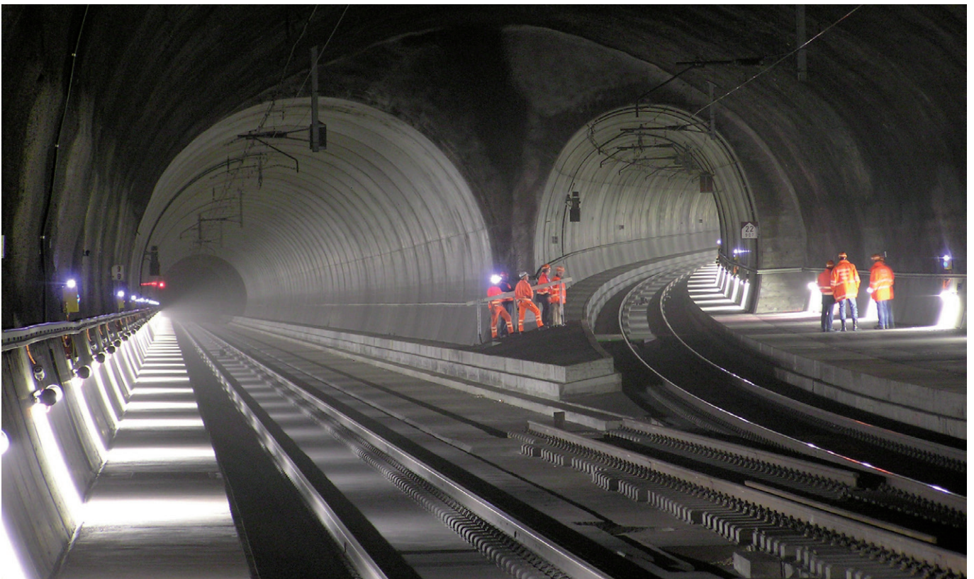
Amelioration of the measurements for self-rescue in the base tunnel Zimmerberg (Zurich – Thalwil)
